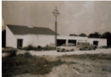
TPC construction in 1976
